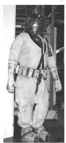
old cumbersome MK5 hard hat rig that many of the members first trained with, and also a new, light weight plastic helmeted hard hat rig that even had provisions for an emergency come home bottle. The new portable aluminum recompression chamber is a great improvement over the old coffin-like portable chamber.
